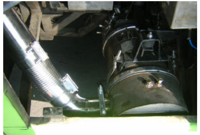
Figure 4. DPF system installed in the bus
