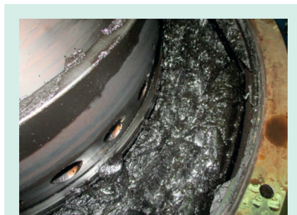
Figure 1. Aged distillates blocking up sludge lines and purifiers; if not removed, this sticky substance can become impregnated with other impurities such as cat fines or sediments, effectively creating a grinding paste inside fuel lines.
